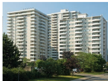
Durand Village in Hamilton is one example of four apartment complexes in Ontario that were retrofitted with water conservation upgrades in 2012.
